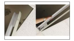
8. From the inside, slide the locking clips under the heads of the M4 screws.
