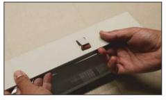
7. Insert the luminaire from below into the mounting adapter. Do not press on the plastic diffuser during this operation!
