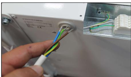
13. Connect the power cable to the terminal block and screw the side cover.
