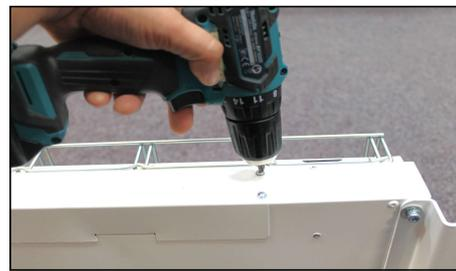
12. Insert the power cable through the rubber grommet into the luminaire.
