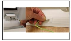
5. Thread the power cable through the membrane grommet and secure the light fixture in place using mounting hardware (not included in the delivery).
