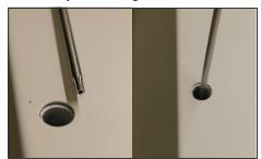
3. Measure and drill holes at the designated location for securing the light fixture.
