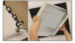
2. The lamp is intended for installation in a suspended ceiling grid with auxiliary suspension
