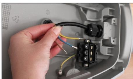
12. Connect wires to the disconnecter.
