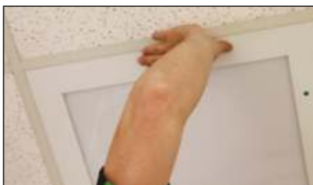
5.2 If necessary, press only on the metal edge
