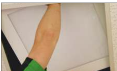
4.2 Place the luminaire in the grid
