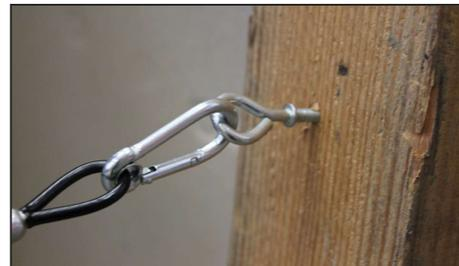
3. Attach the luminaire fixture to the designated location using a suitable connecting material.
