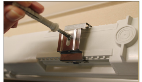
6. Fasten the clips to the substrate in the given spacing of mounting points on the light fixture
