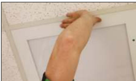
5.2 If necessary, press only on the metal edge
