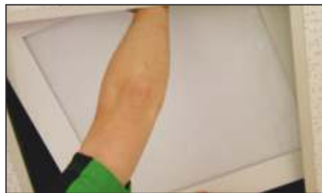
4.2 Place the luminaire in the grid
