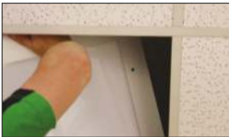
4.1 After connecting the power cable, slide the lamp diagonally into the ceiling.
