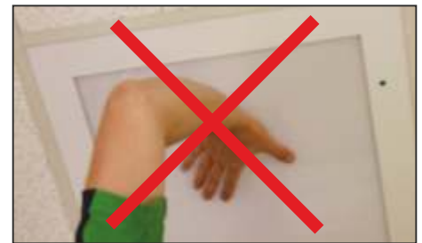
5.1 When handling the lamp, do not press on the plastic diffuser
